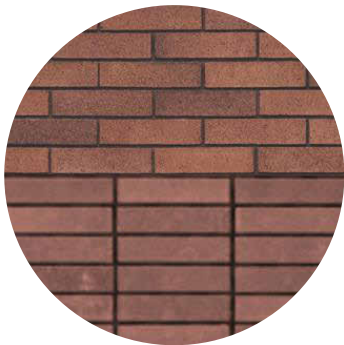
8. BRICK - RUNNING & STACKING BOND * (PART OF S4.55 APPLICATION)
